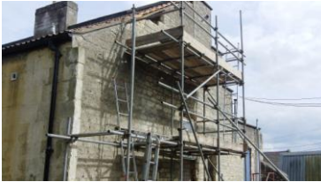
Bradford on Avon repair in progress ...
