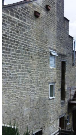
... and repair complete.
